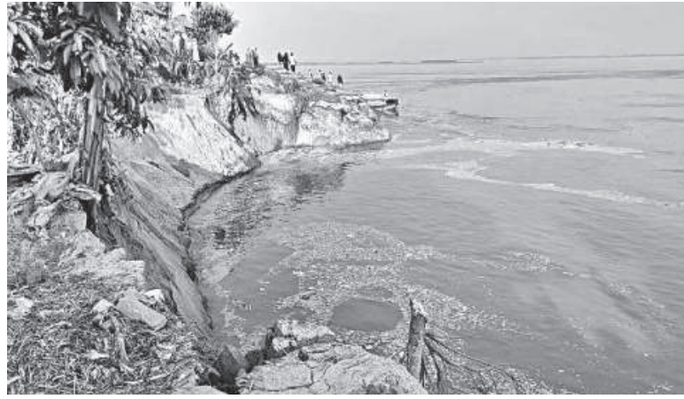
Erosion along 150 metres of the Jamuna river in Chongacha union of Sirajganj devoured at least 20 homes, while displacing over 30 families recently.
