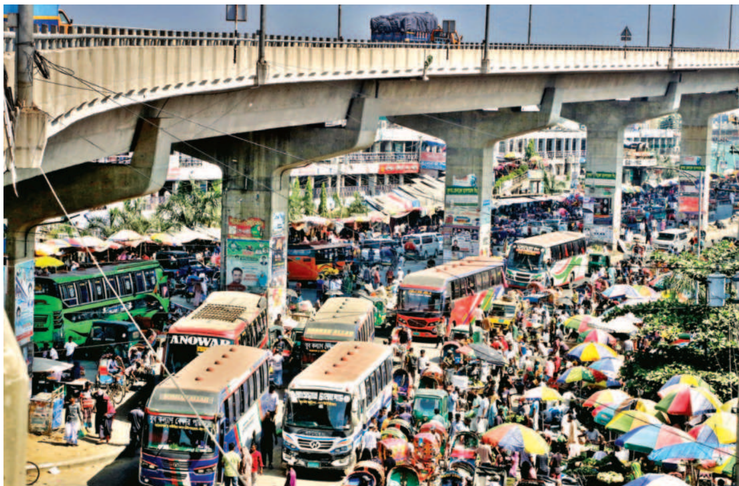
Vehicles struggling to pass the area under the Bhulta overpass in Narayanganj's Araihaazar, as a make-shift bazar has sprung up there, occupying a portion of the Dhaka-Sylhet highway. The authorities have turned a blind eye to the problem. The photo was taken yesterday.
