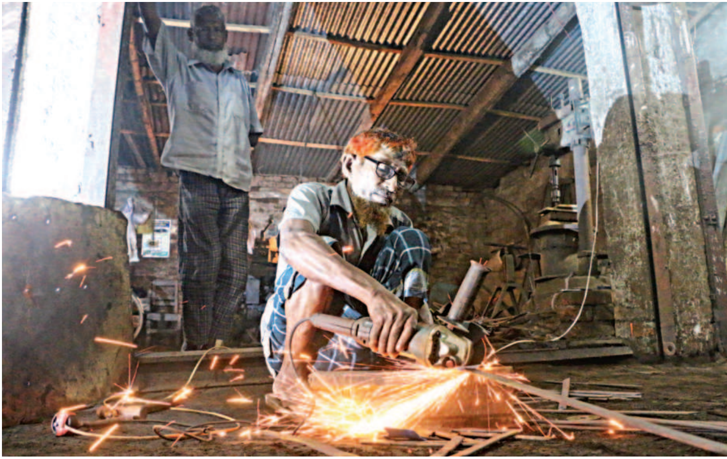
Md Akbar Ali cuts strips of metal to create window grilles at his workshop in Bagachra union of Jashore. He purchases each kilogramme for Tk 97 to Tk 98 and sells the final product, be it gates, shutters or window grilles, based on the weight at Tk 125 to Tk 130 per kilogramme. He charges just Tk 28 to Tk 30 per kilogramme for the use of his craftsmanship gathered over the past 44 years. Bangladesh currently requires 80 lakh tonnes of steel and in terms of annual sales, the size of the market is about Tk 72,000 crore as per the current rates, according to industry operators. The photo was taken last week.
