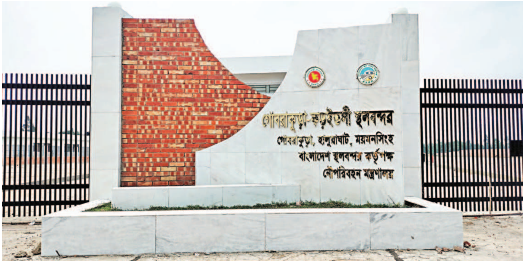
With all development works now complete, the Gubrakura-Karaitali land port in Haluaghat upazila of Mymensingh will begin operating at full capacity from next month.
