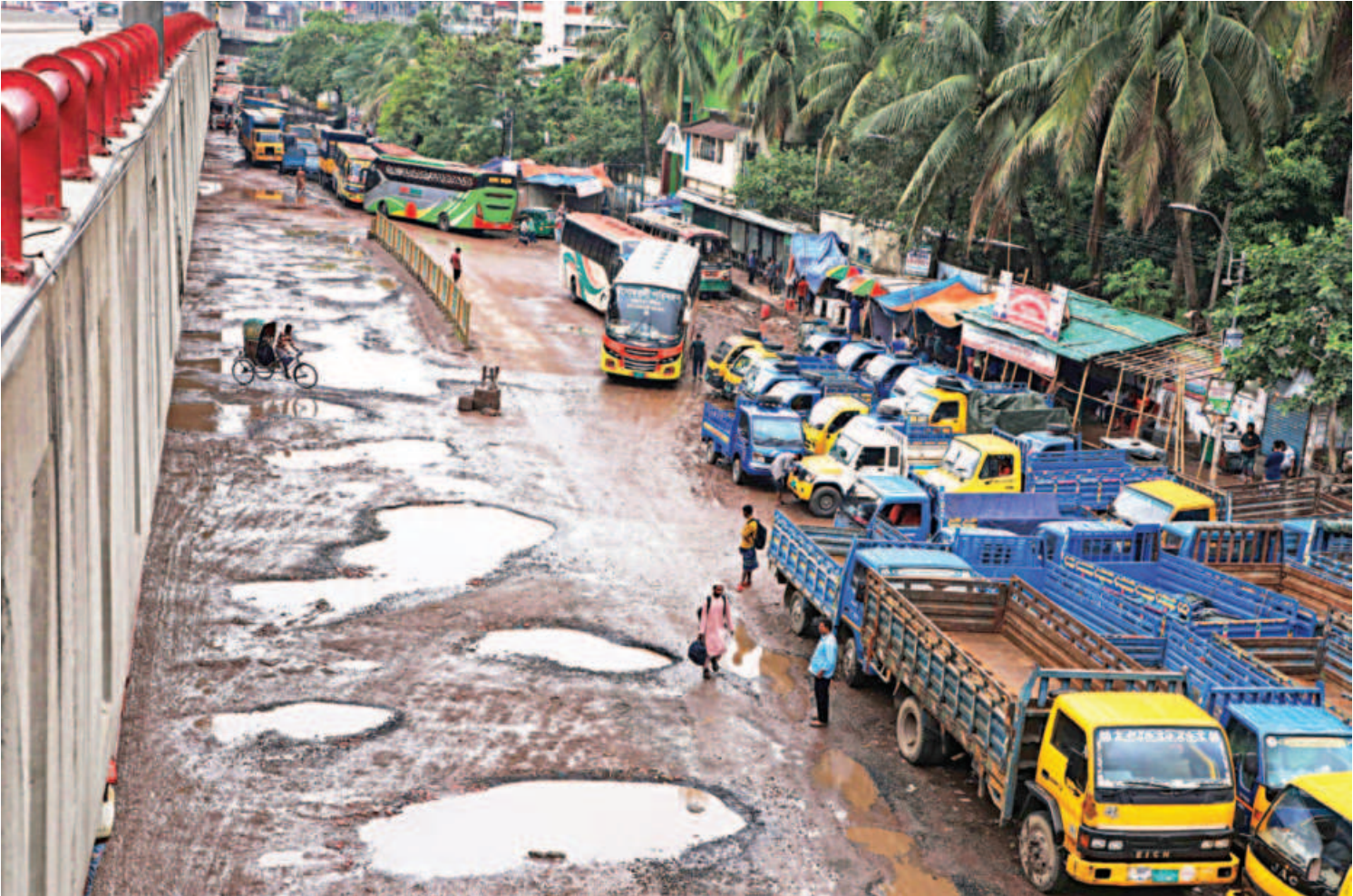
A section of the Dhaka-Chattogram highway beneath the Mayor Hanif Flyover near Jatrabari intersection are littered with crater-like potholes, which are deep enough to even topple vehicles. The other side of the road is occupied by illegally parked trucks. The photo was taken yesterday.
