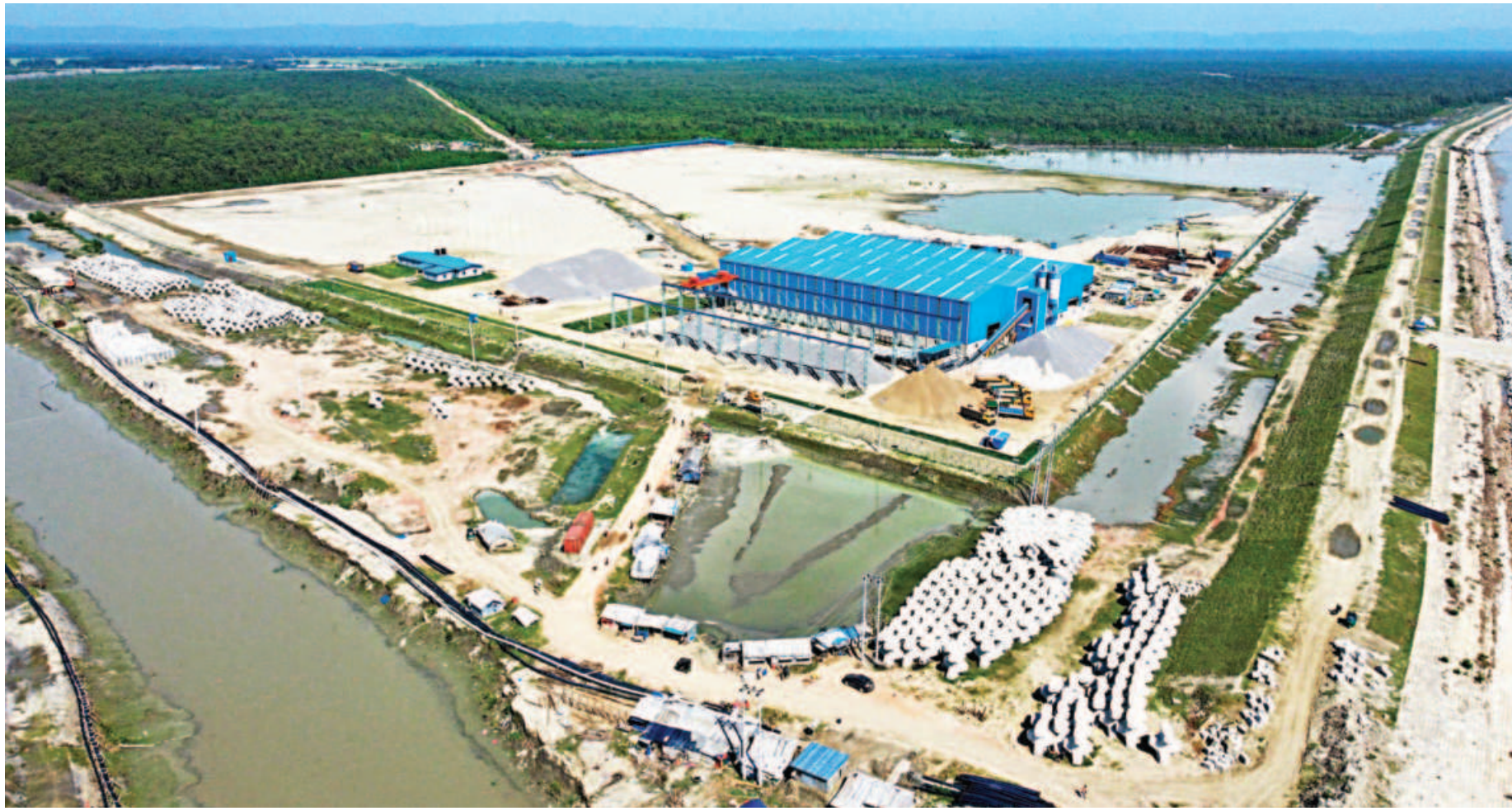
The Bangabandhu Sheikh Mujib Shilpa Nagar being developed on 33,000 acres of land in Chattogram is shaping up to be the largest industrial enclave in the country. As such, the Bangladesh Economic Zones Authority has assured that utility services will be provided on a priority basis for investors, who have already poured considerable funds into the project.
