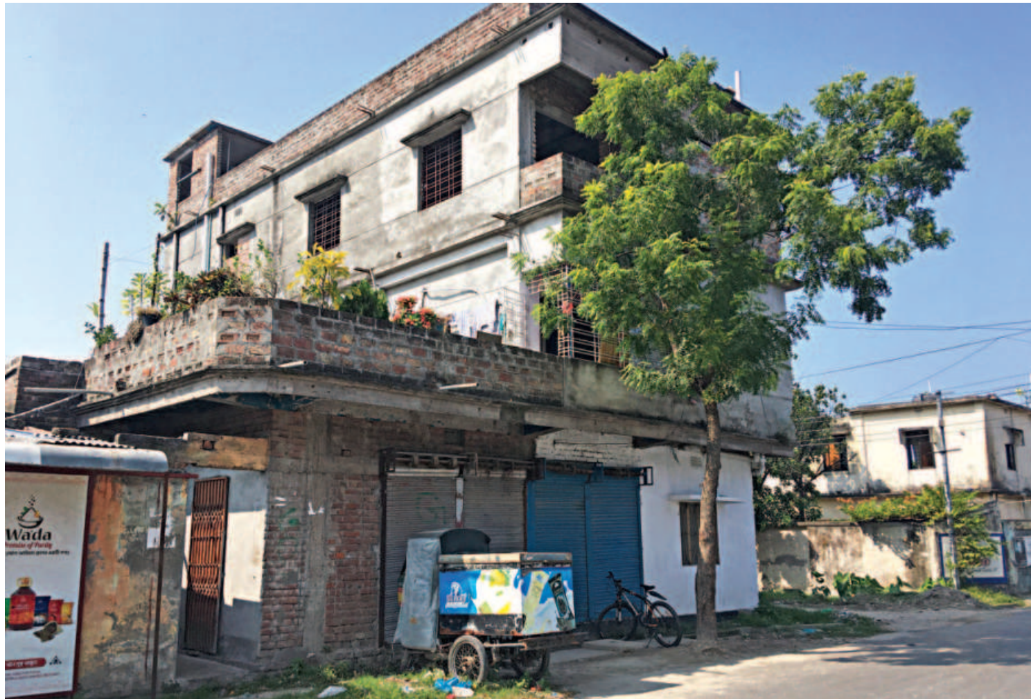
The Keramat Rice Mills situated on two plots inside the BSCIC industrial estate in Rajshahi seems more like a ramshackle apartment complex than an industrial unit as its owners have long been renting it out as such. Following repeated warnings from the estate authorities, the residents have set up small-scale light engineering units to allay concerns.
