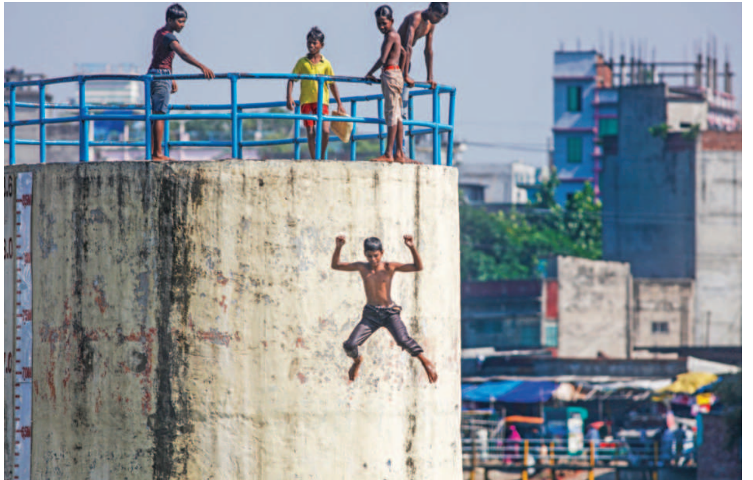
Even though this water measurement pillar is situated in the middle of the river, local children, evading the rules, get on top of the structure and take a dive into the river for fun. Such "playful" activities can lead to a serious accident. This photo was taken in Kamrangirchar area yesterday.
