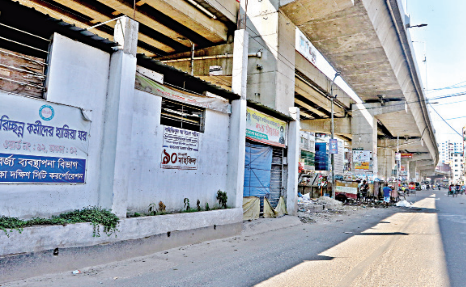
Underneath the Moghbazar-Mouchak flyover, the city corporation has set up a “secondary transfer station” for proper waste management. However it has been turned into an office for cleaners where waste collection vans are kept. As a result, garbage is still being dumped beside the station after collecting those from households. The unloading of garbage from vans not only leads to traffic jams, pedestrians also have to deal with a residual odour of rotten items. This photo was taken near the Malibagh Rail Crossing area yesterday.
