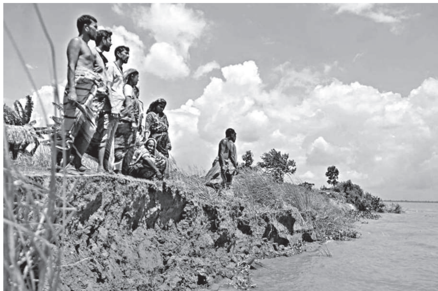
Looking out to the distance, residents in Faridpur Sadar have only one thing in their mind -- "Where will we go now?". Many have lost their homes twice now due to the erosion caused by the Padma. With no sustainable solutions in sight, they silently mourn their lost homes.
