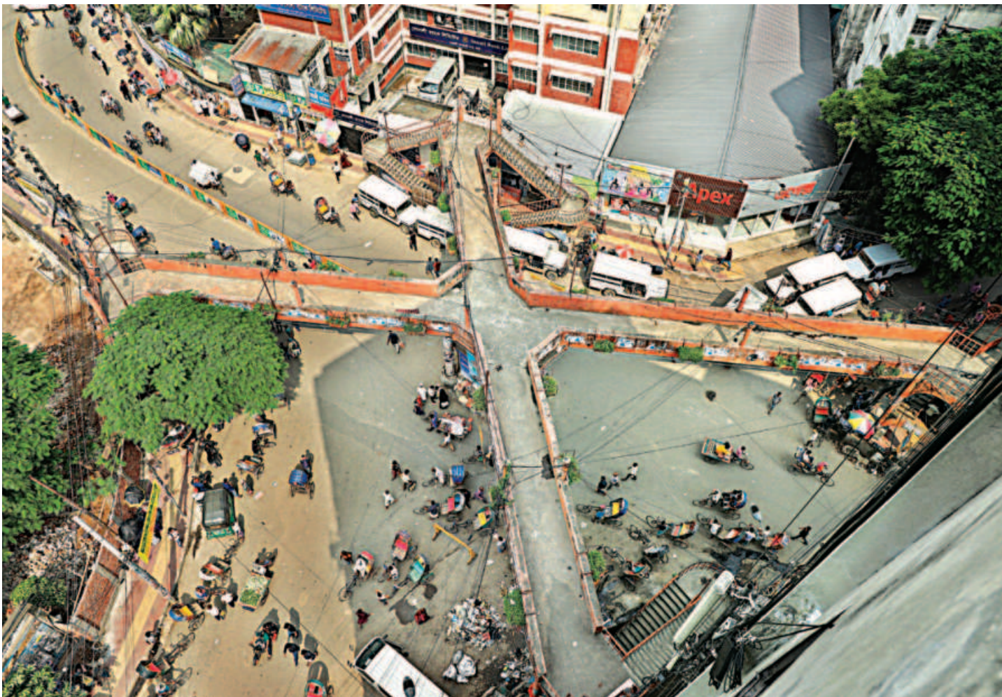
An empty footbridge at Banglabazar intersection in the capital as pedestrians would rather jaywalk than climb a flight of stairs. The photo was taken yesterday.
