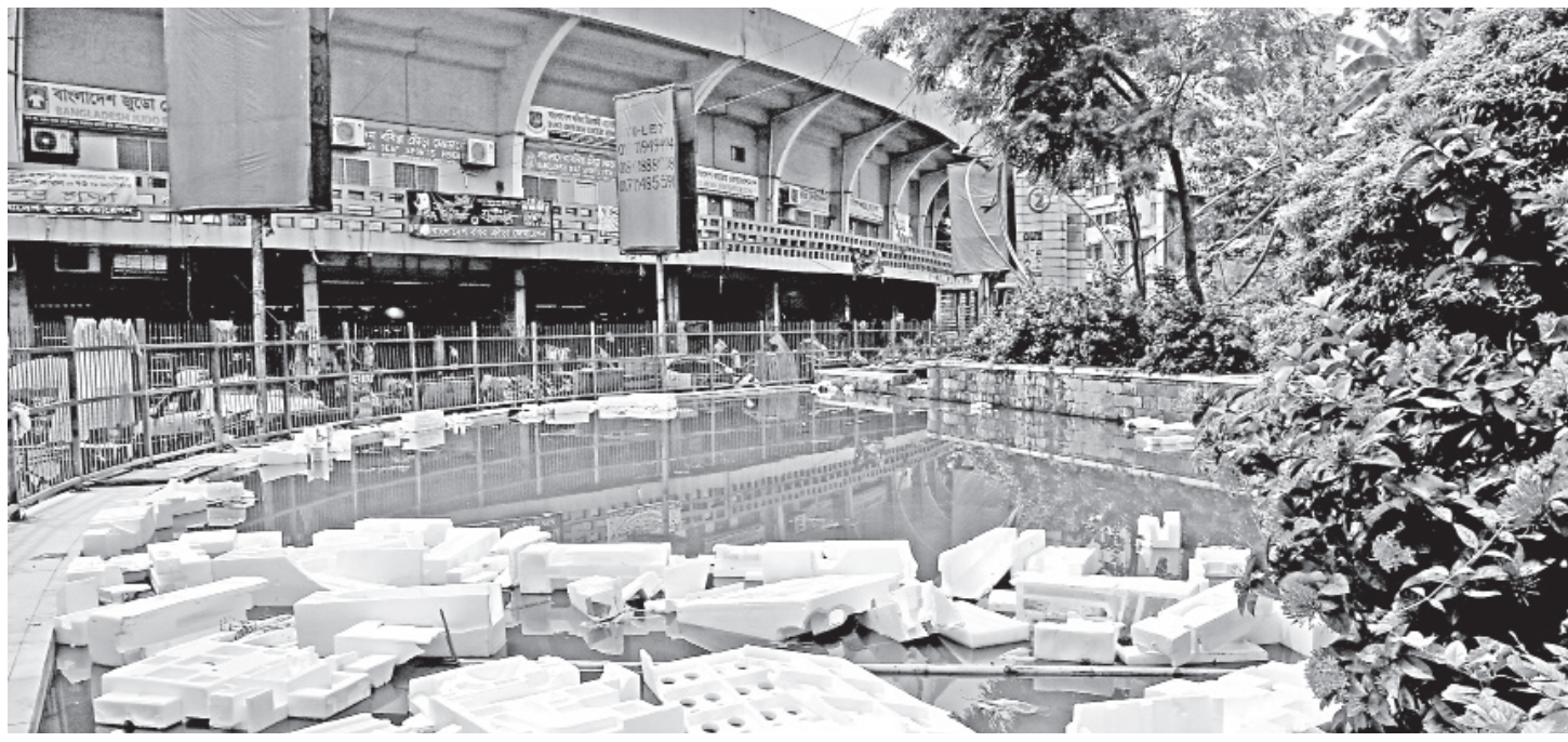
Although this structure at the heart of the capital's Bangabandhu Stadium was meant for beautification, lack of maintenance has turned it into an eyesore. Meanwhile, owners of nearby shops continue to dump cork sheets received in the packaging of different products there. This photo was taken in Gulistan area recently.
