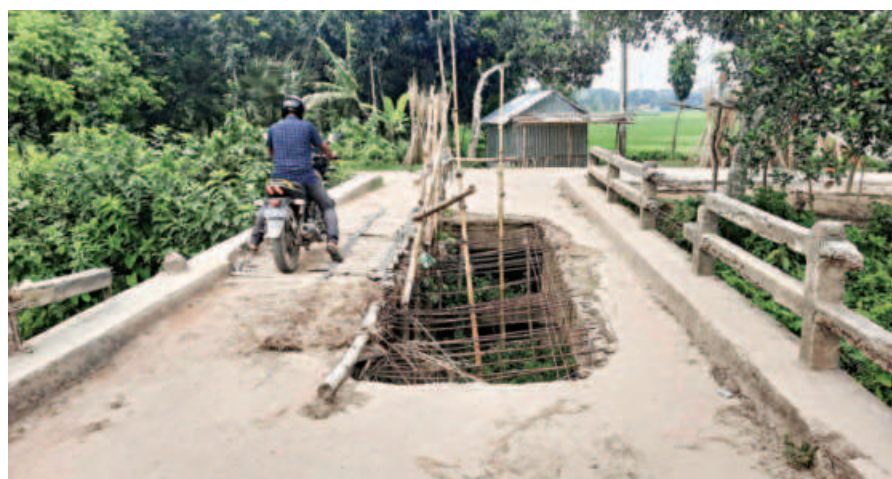
Part of the deck of this bridge on Alamdanga Canal in Jhenidah's Shailakupa upazila remains unrepaired for years, making it difficult for vehicles to cross it.
