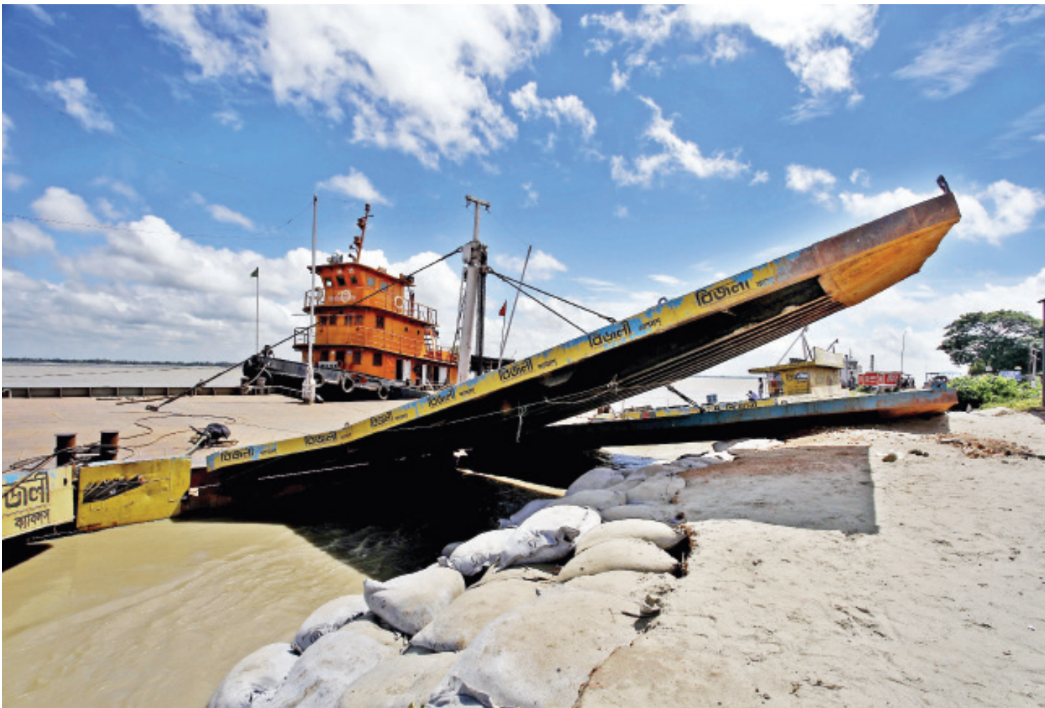
A pulled up ramp of a pontoon at Daulatdia Ferry Terminal in Rajbari as recent erosion of the banks of the Padma have rendered this and several pontoons unusable. The photo was taken yesterday.
