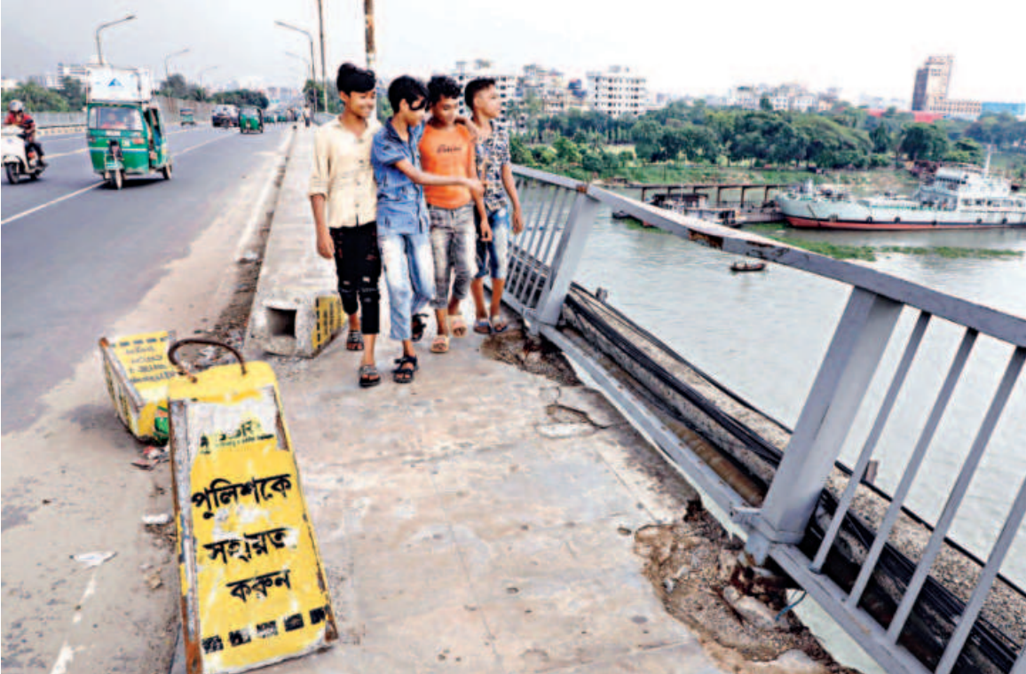
Friends taking an afternoon stroll is a common scene on the Postogola Bridge. However, a part of the railing was damaged after an accident and has been left unfixed by the authorities concerned for a while now. A moment’s lapse could turn this enjoyable walk into a tragedy. This photo was taken yesterday.
