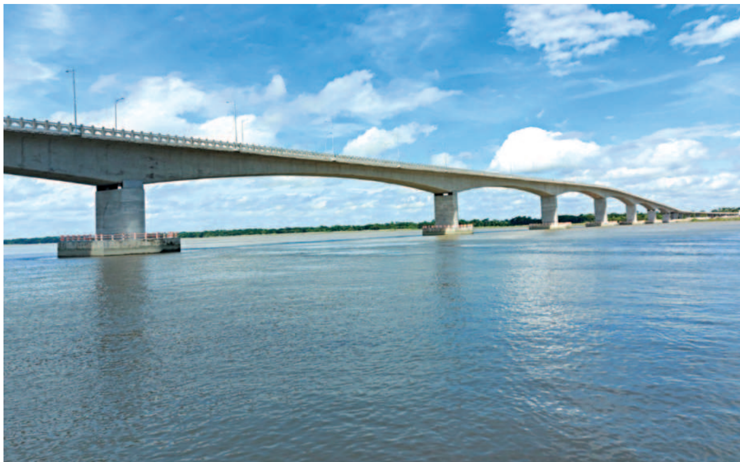
The long-cherished Bekutia bridge on the Kacha river in Pirojpur is set to be inaugurated today by Prime Minister Sheikh Hasina. The 1.49km structure, officially named Bangamata Begum Fazilatun Nesa Mujib 8th Bangladesh-China Friendship Bridge, will establish direct road link between Barishal city and Pirojpur. The photo was taken recently.
