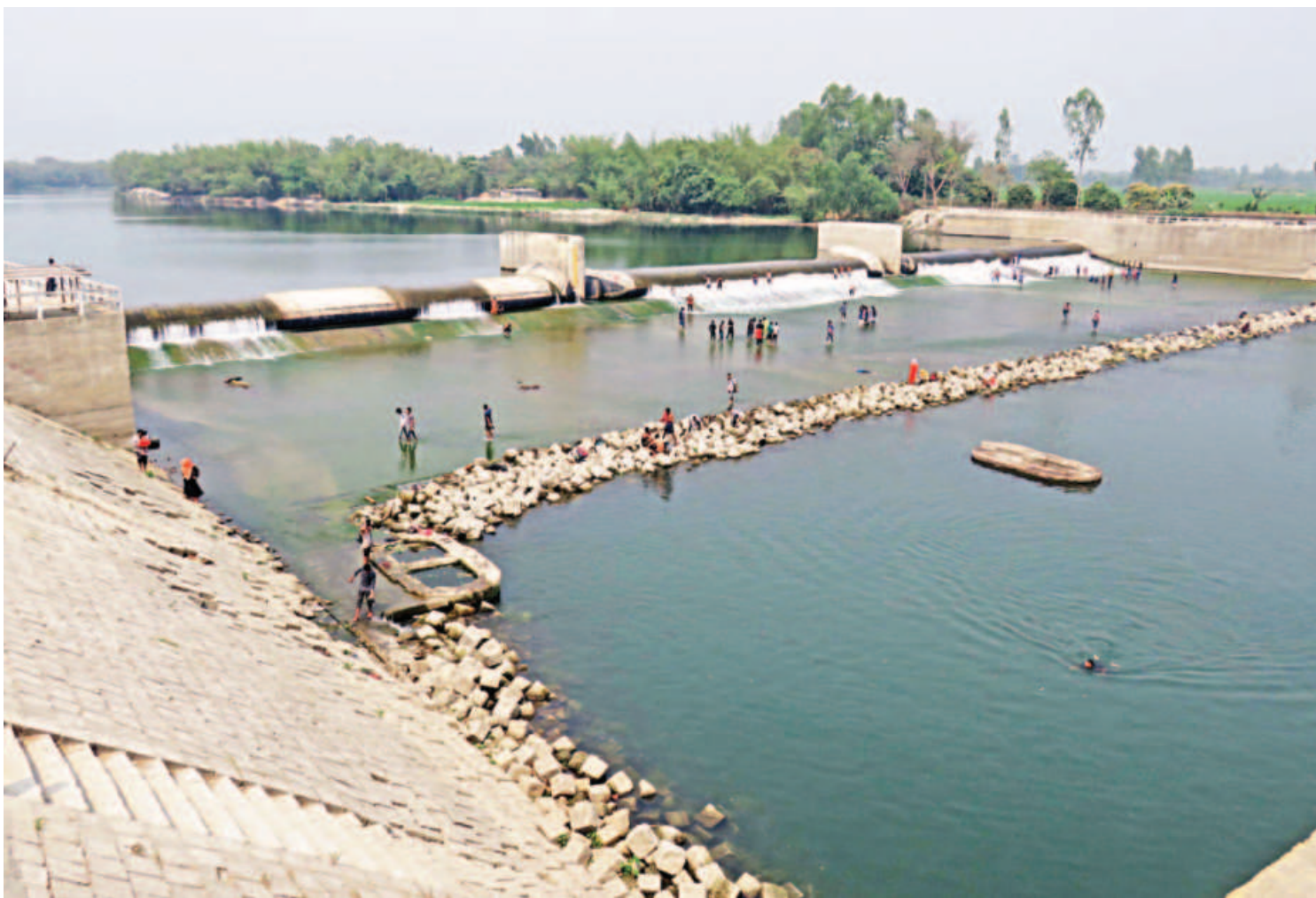
This rubber dam on the Atrai river ensures that farmers in six unions across Dinajpur sadar upazila and Chirirbandar upazila have enough water to irrigate their fields year-round. The use of surface water for irrigation is rising amid depleting underground reserves and higher extraction costs.
