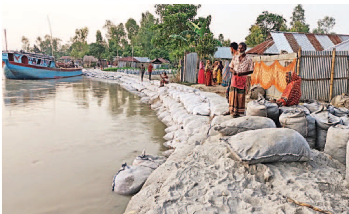
WDB dumping sand bags in different erosion-hit areas to protect the river banks. The photo was taken from Purbo Kalmati village in Lalmonirhat Sadar upazila.
