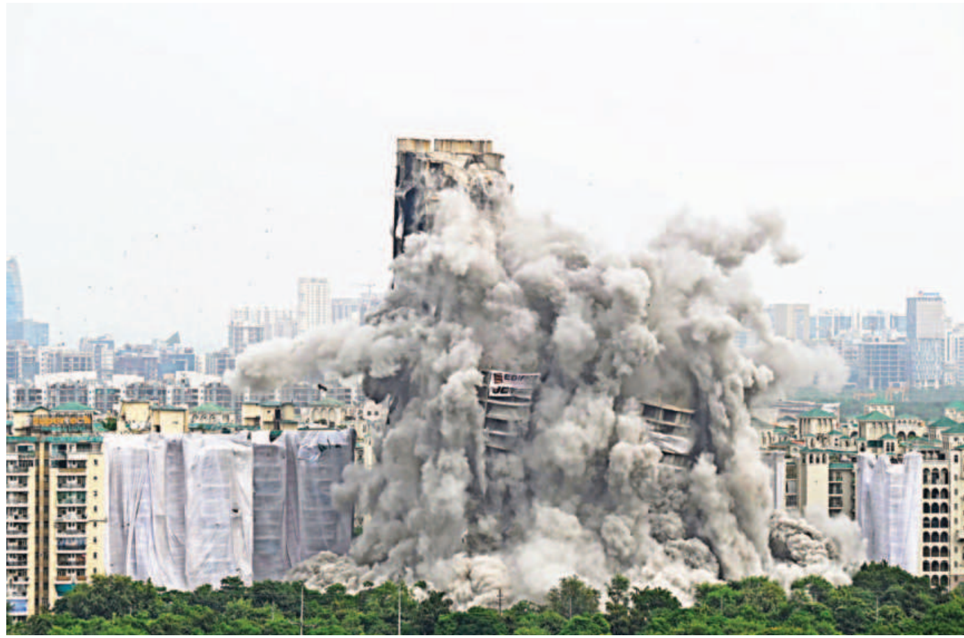
A controlled implosion demolishes the 100-metre-high residential "Twin Towers" in Noida on the outskirts of New Delhi, yesterday. Two illegally built residential high-rises were demolished near India's capital in a rare crackdown on developers who cut corners and swindle unsuspecting home-buyers. PHOTO: AFP
