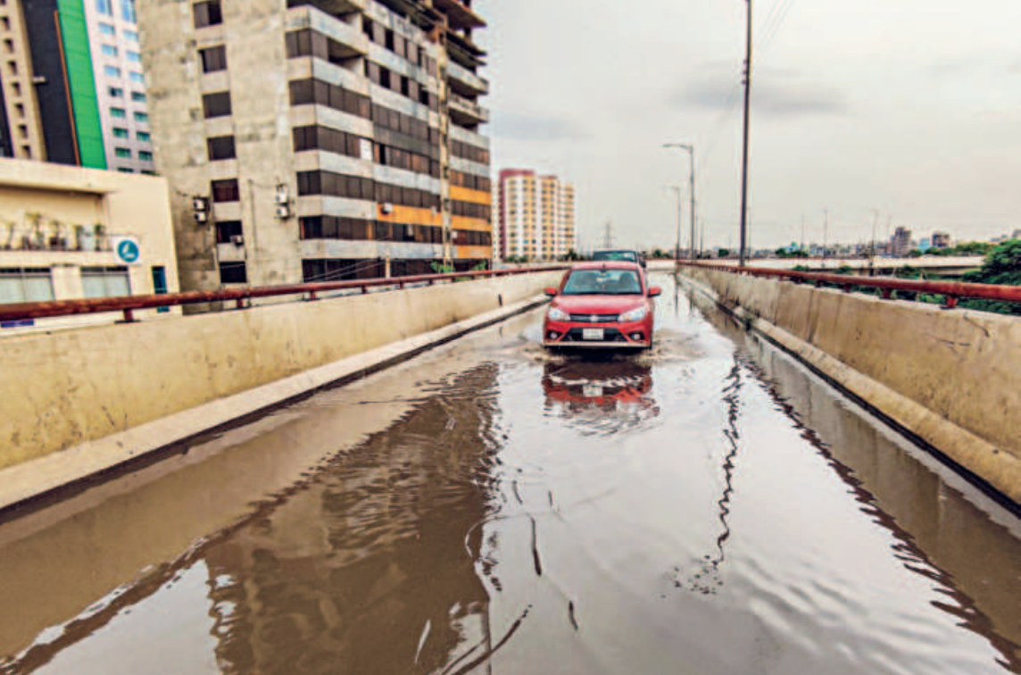
A car slows down while crossing a waterlogged part of the Moghbazar flyover yesterday. Due to a lack of maintenance and proper planning during construction, water accumulates in the flyover, even after a slight drizzle.
