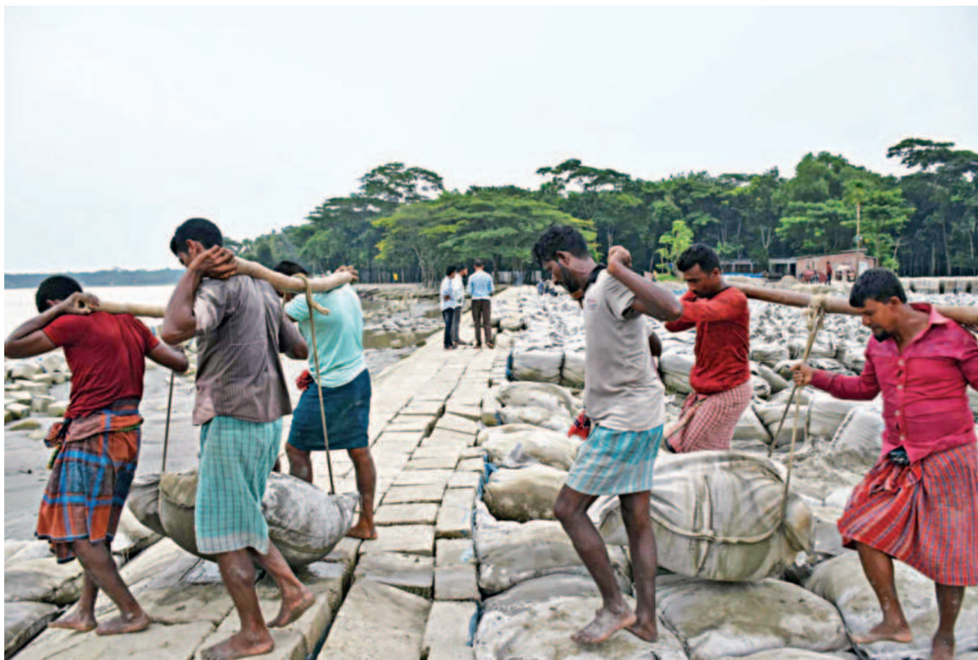
Sandbags being taken to the Kirtankhola to protect its banks from erosion. Labourers who are carrying these bags earn between Tk 500 and Tk 800 daily. The photo was taken in Barishal Sadar upazila yesterday.
