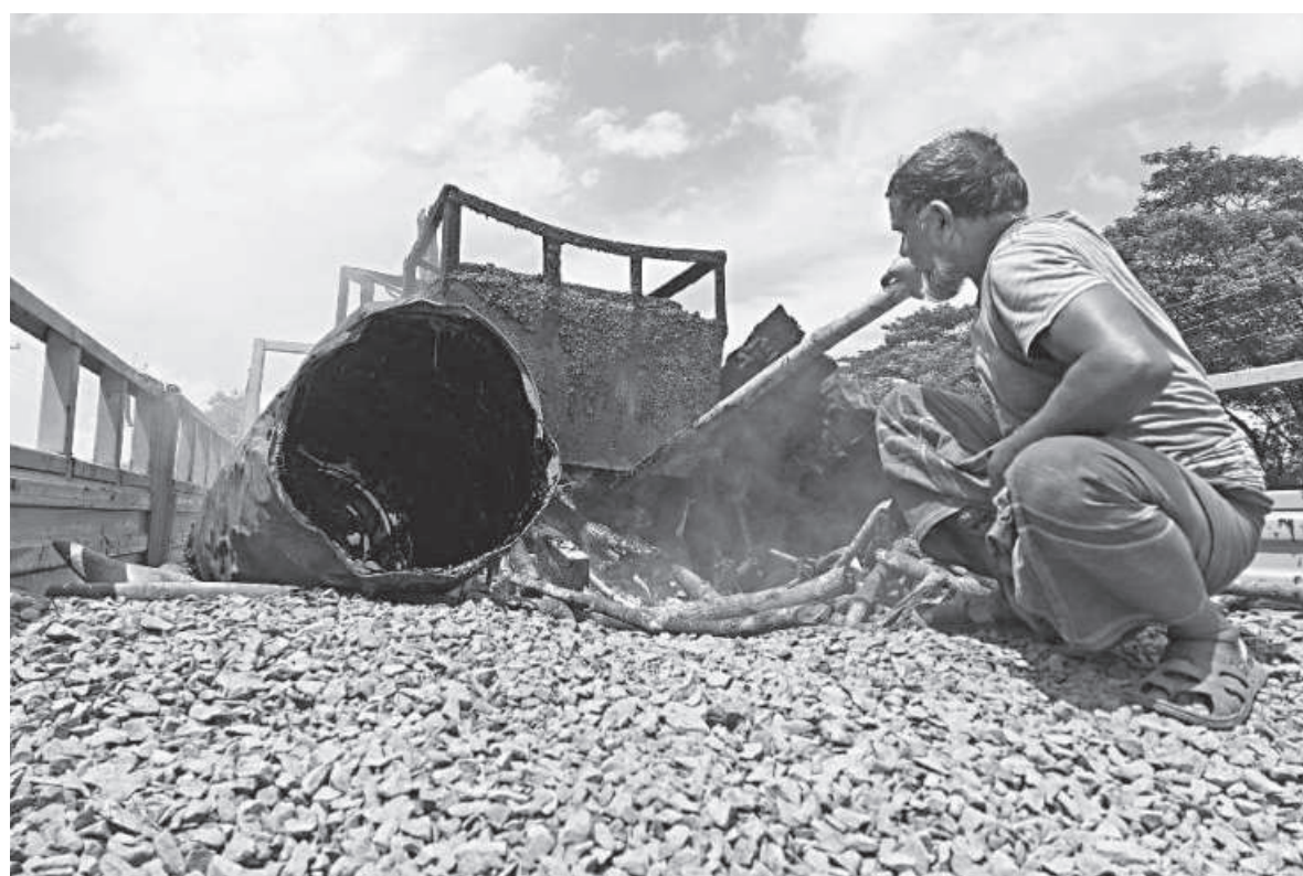
A worker melting pitch in a boiler machine for emergency repairs of potholes on Barishal-Dhaka highway. This photo was taken in Rahmatpur area of Barishal's Babuganj upazila. PHOTO: TITU DAS
