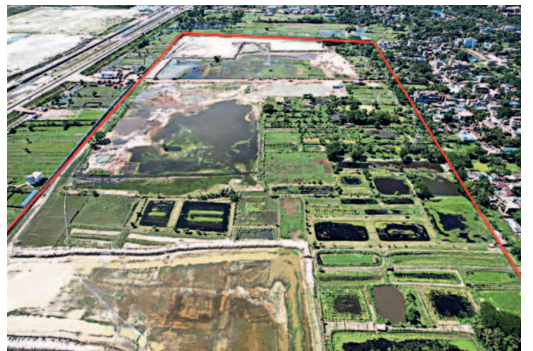
The allocated land for the Sewerage Treatment Plant (STP) of Chattogram Water Supply and Sewerage Authority.
