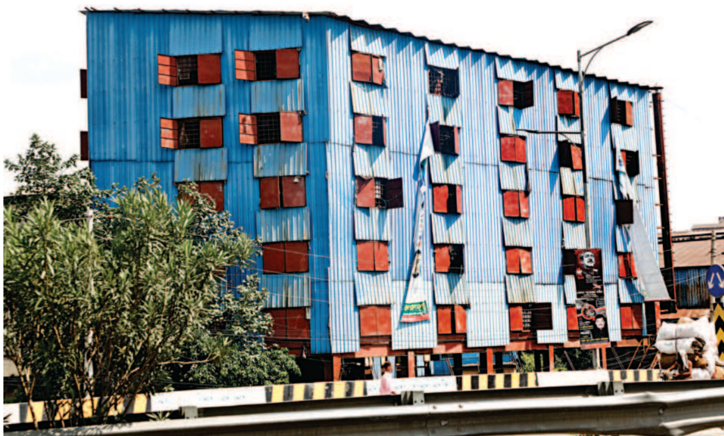
While passing by Postogola area yesterday, this photojournalist came across a rather odd, five-storey tin structure, where labourers of nearby re-rolling mills live. Although it seems to be standing tall for now, it is still doubtful whether this structure even passes the basic fitness check.
