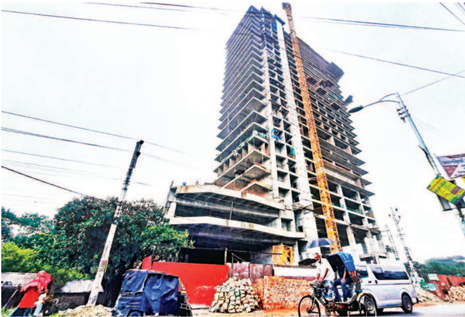
A multistorey building under construction right by the Khulna-Jashore road at Boikali Mor in Khulna city, devoid of safety measures such as nets to protect passers-by from falling objects. The photo was taken recently.
