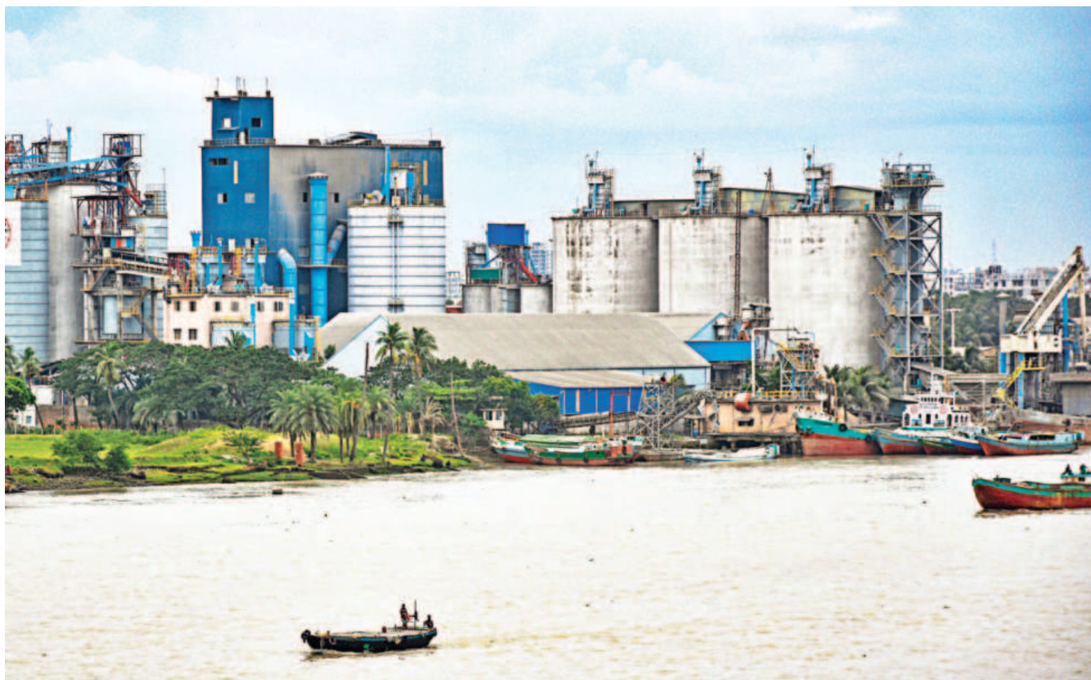
A cement factory by the Rupsha river in Khulna. Cement production grew just 0.26 per cent year-on-year to 1.79 crore tonnes in the last 10 months till April, according to the Bangladesh Bureau of Statistics. Industry insiders see a dearth in demand because of the government's austerity measures and the private sector's cautious stance in taking new construction projects.
