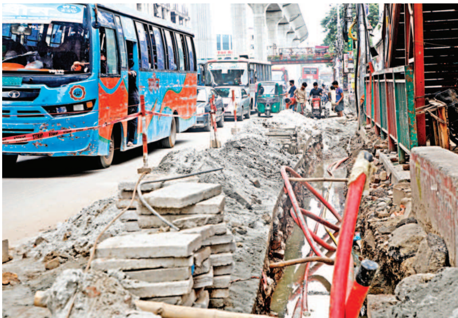
As part of development works, the authorities have dug up a side of the busy Kazi Nazrul Avenue near Karwan Bazar and kept it that way for a while. As work progresses slowly, the biggest sufferers are the commuters, who have to push through gridlock every day while traveling on the road. This photo was taken recently.
