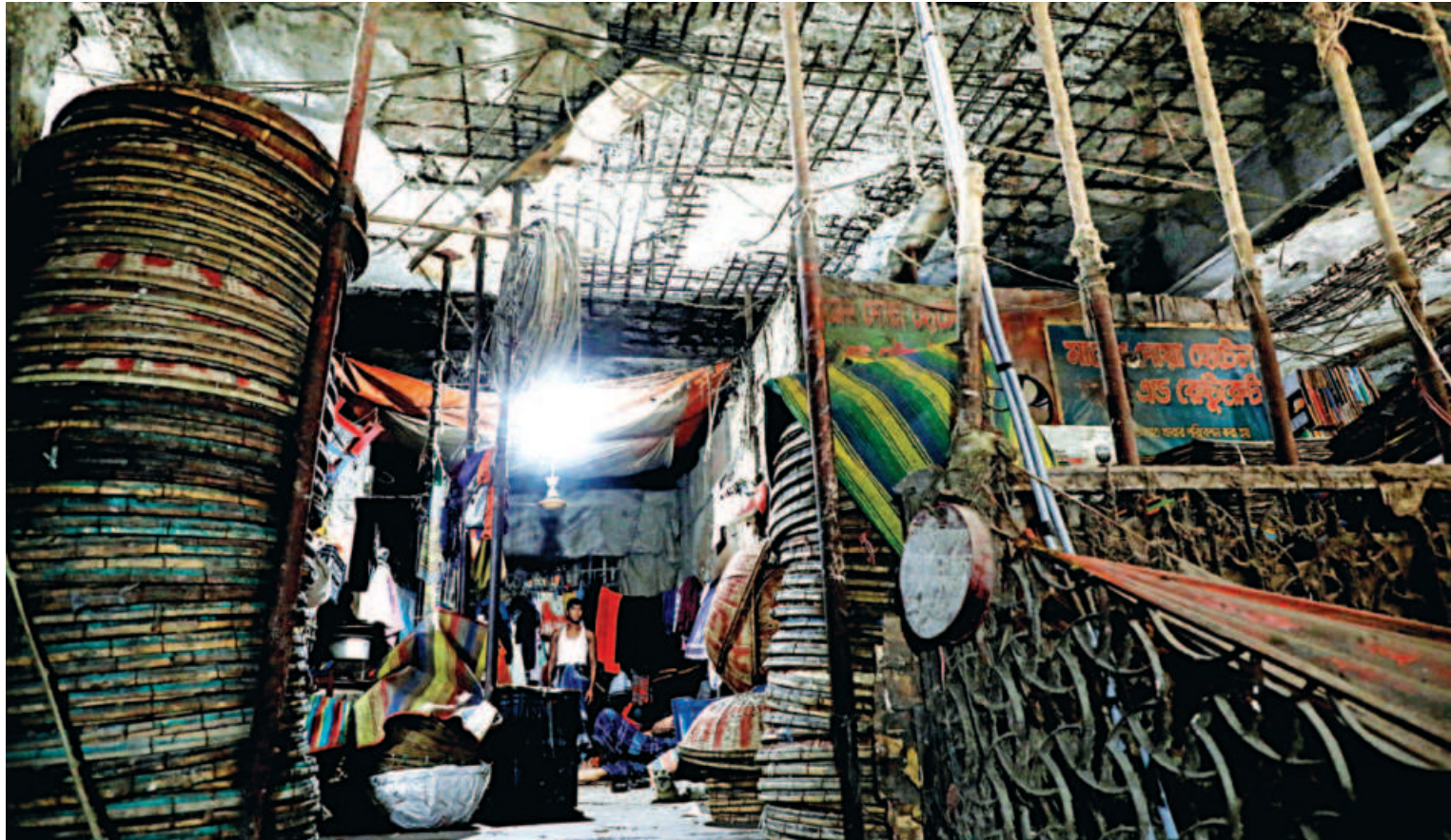
The ramshackle Paka Arot Bhaban of the capital's Karwan Bazar is in danger of caving in any time. The roof of the building has been propped up with iron pipes to avoid collapse. Traders still run businesses there, putting themselves and customers in harm's way. The photo was taken yesterday.
