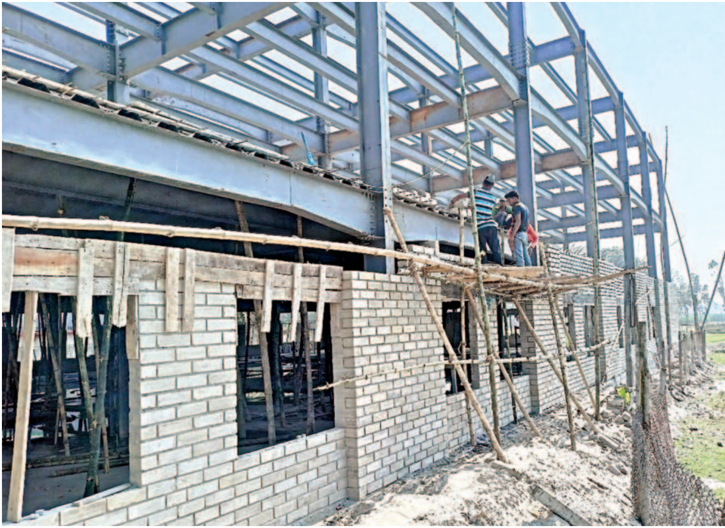
Workers are seen fitting eco-friendly concrete blocks into place at the construction site of an export-oriented handicraft factory in Nilphamari. These blocks are made from sustainable materials such as fly ash and do not require baking in kilns unlike their traditional counterpart.
