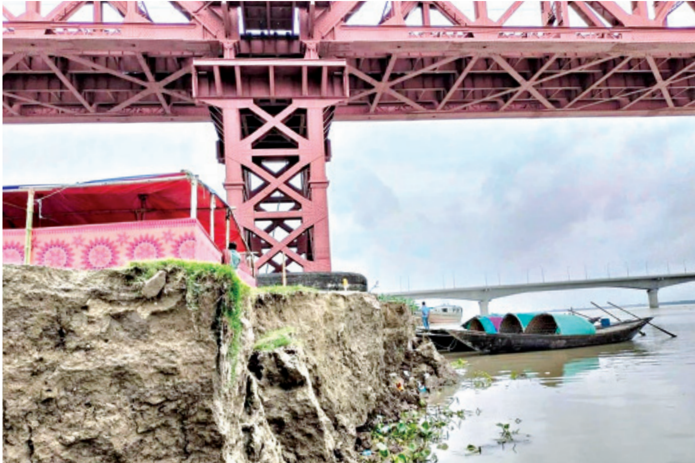
River erosion eating away riverbanks at the Sara and Rooppur points of the Padma, where the Hardinge Bridge, the oldest rail bridge in the country, stands. Railway officials claimed the erosion is unlikely to harm the bridge but they are observing the situation. The photo was taken near the bridge's girder-2 in Pabna's Pakshey upazila recently.
