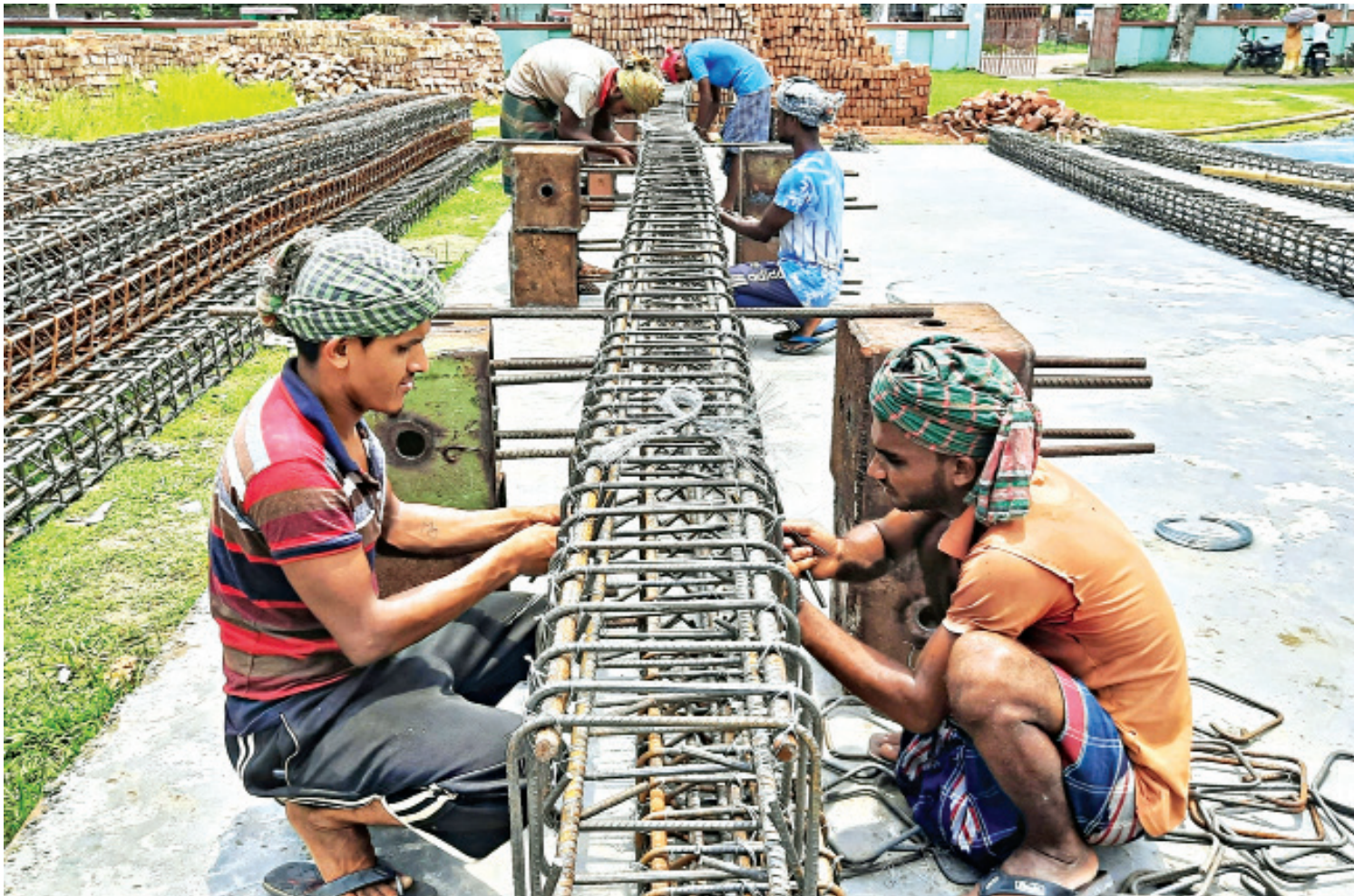
Workers construct frames out of metal rods and wires for use in the piling process of high-rise buildings. Working together from sunrise to sunset, they can make 10 such frames of 50 feet each, earning Tk 550 per person. The photo was taken recently.
