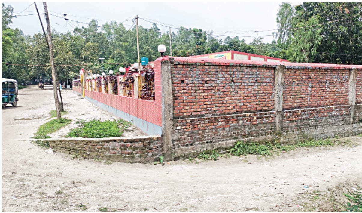
A local ruling party leader built this illegal establishment on Water Development Board (WDB) land just beside the flood bypass road at Doani in Lalmonirhat's Hatibandha upazila. PHOTO: S DILIP ROY
