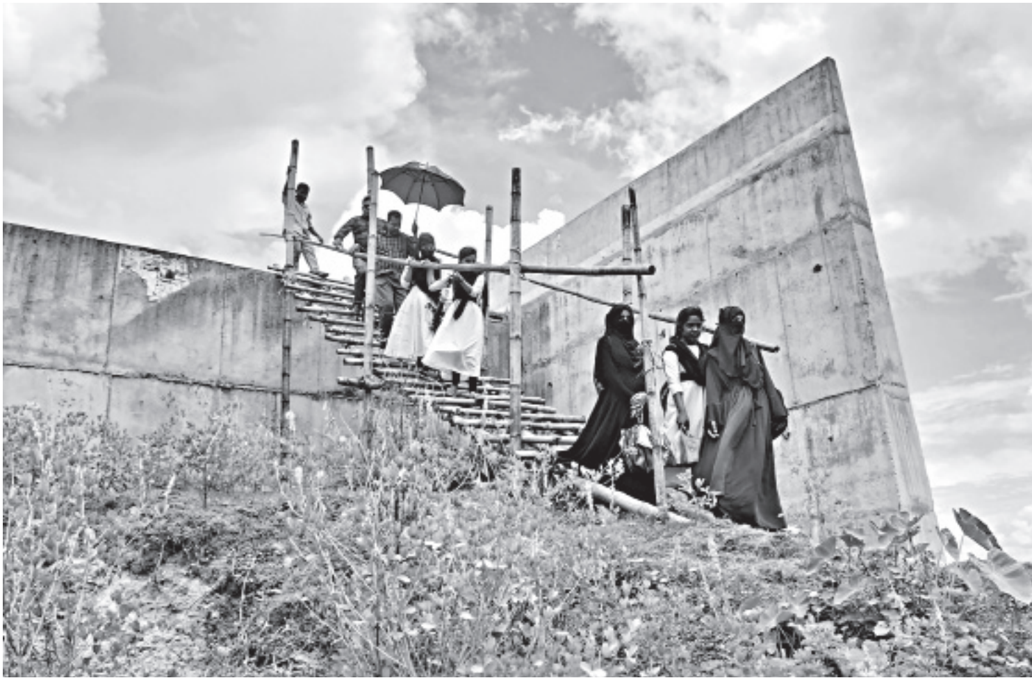
Even though Rajapur bridge over the Manu river in Moulvibazar was built to ease locals' commuting hassle, in reality, it is far from serving that purpose. The connecting road required to make the bridge functional is yet to see the light of day. As a result, people are using steep bamboo platforms on both sides of the bridge, risking their lives just to get across.
