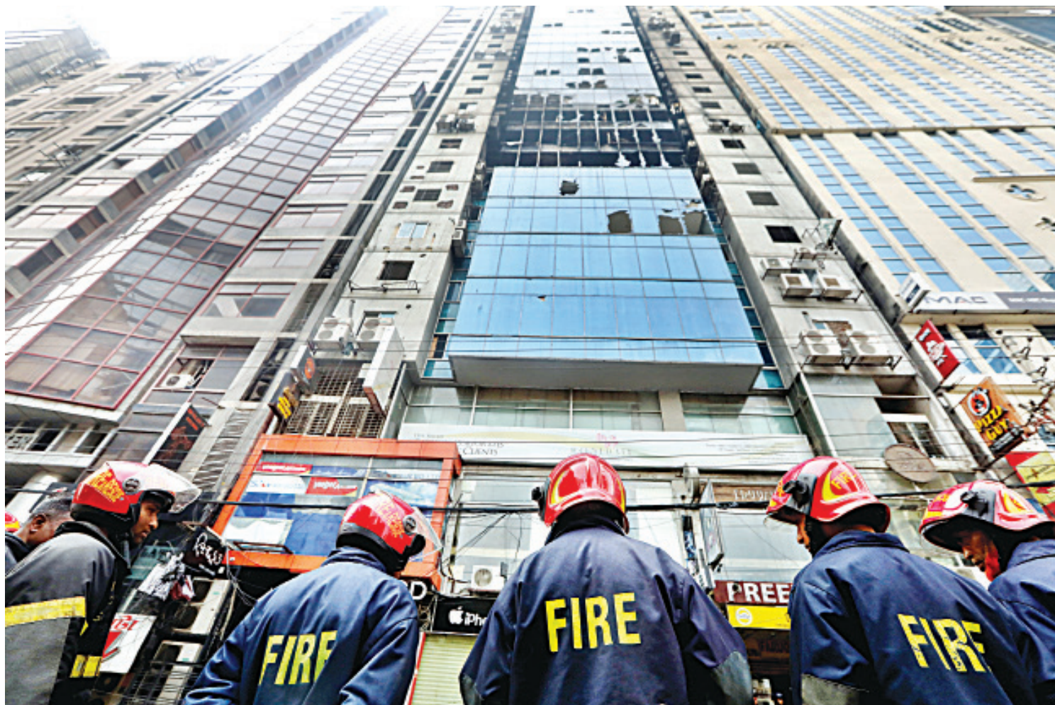
An analyst says there is no scope to delay the construction of public interest projects such as fire stations as this kind of delay may intensify the loss of properties and human lives.
