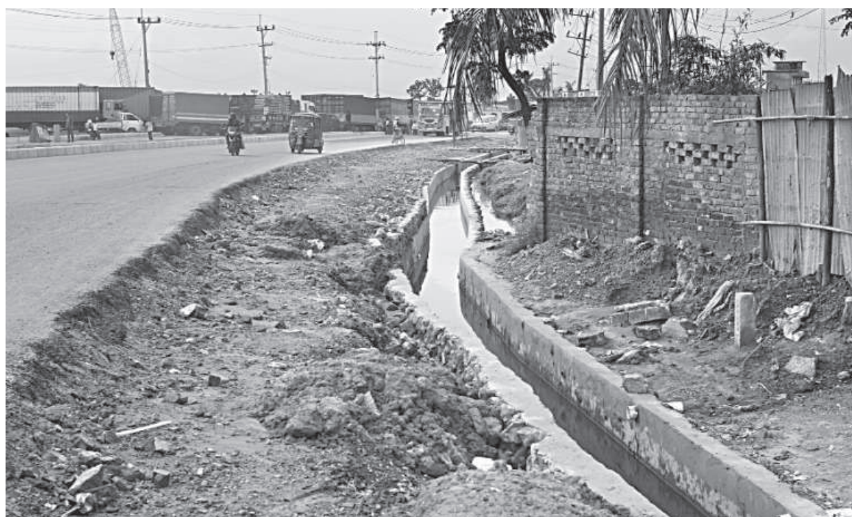
This is the present state of this part of Golden Beach canal in Patenga. The waterway that is supposed to be 60 feet wide is now just like a drain. Karnaphuli tunnel authorities have narrowed the canal -- despite city corporation's objections -- to widen the adjacent road. This photo was taken yesterday. PHOTO: STAR
