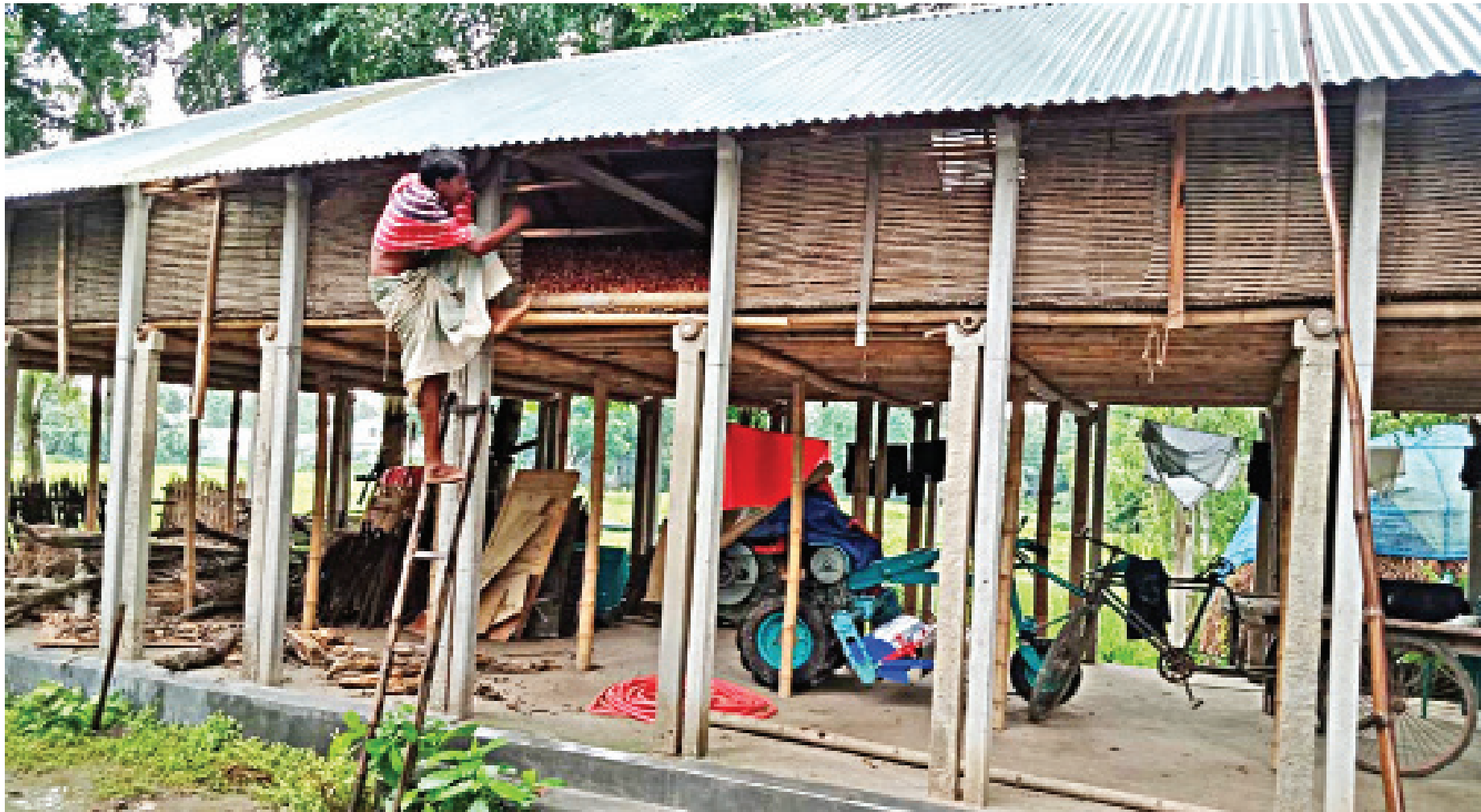
Onion farmers are forced to erect bamboo lofts such as this outside their homes in order to store their produce year-round due to a lack of modern facilities. However, the rudimentary design of these shacks means that the bulbs stored inside are susceptible to adverse weather conditions.
