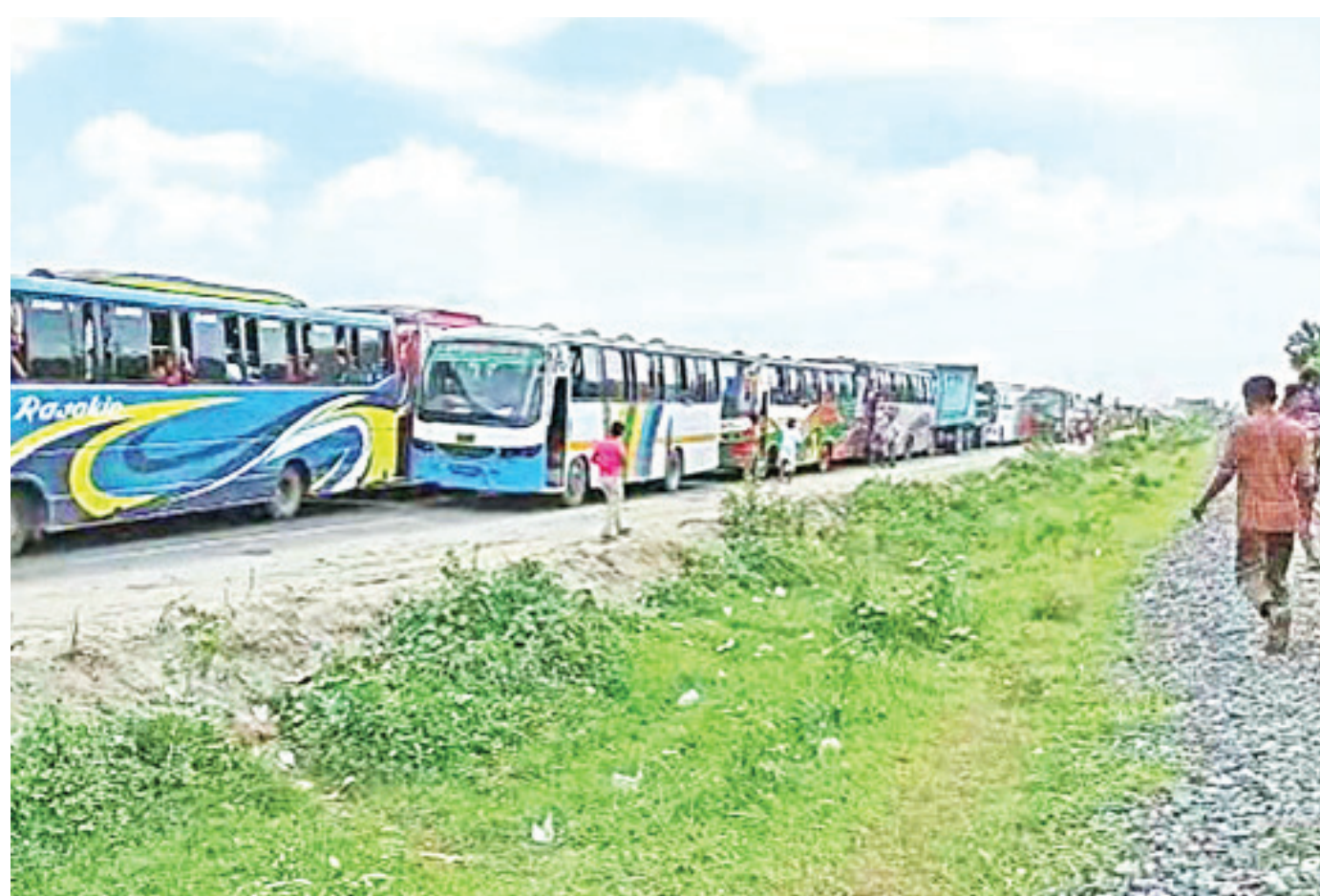
Vehicular movement on Bangabandhu Bridge's east approach road in Tangail has been almost standstill yesterday due to heavy traffic and a truck flipping over. People returning to Dhaka after Eid holidays waited hours in the heat. The photograph was taken yesterday afternoon.
