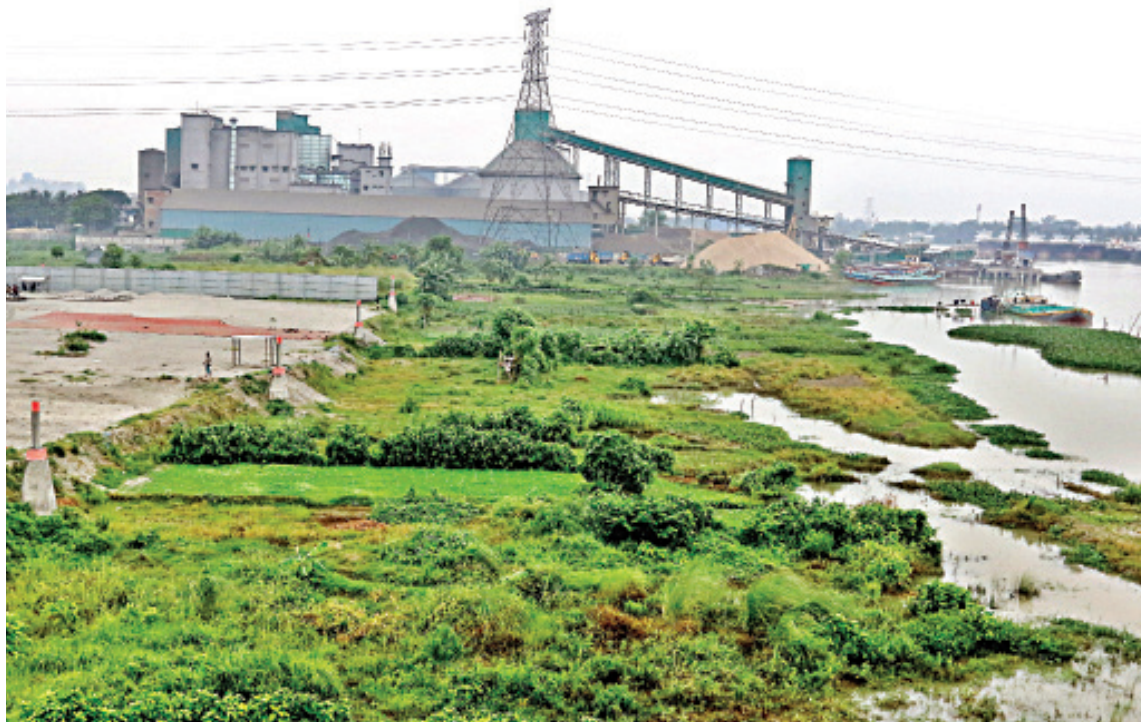
Land grabbers have encroached on the Shitalakkhya in Ichakhali area of Narayanganj's Rugganj, narrowing down the river. The photo was taken recently.
