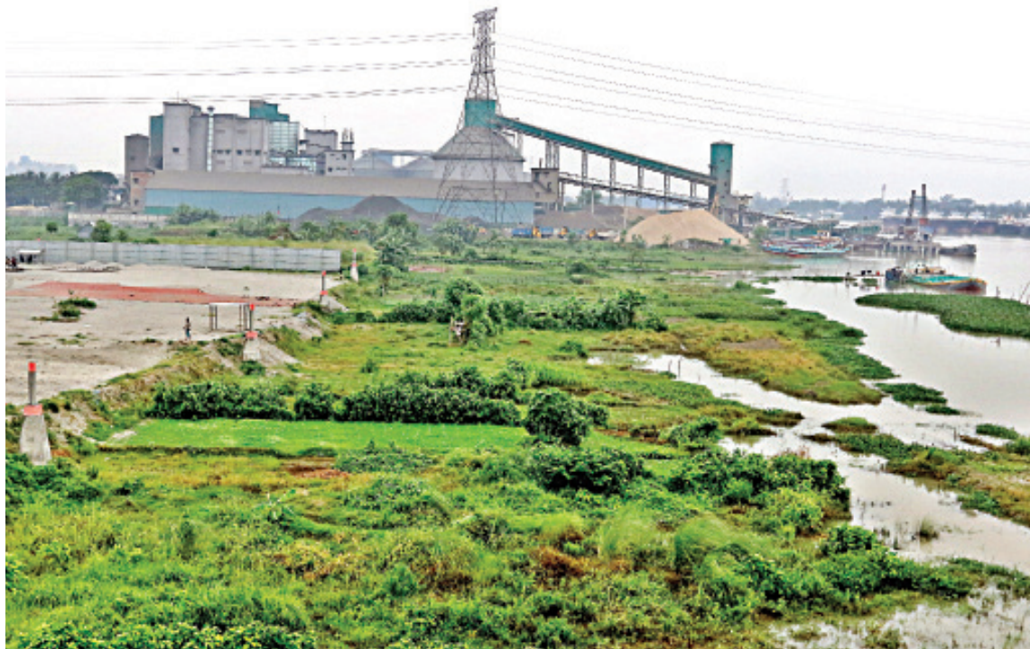
Land grabbers have encroached on the Shitalakkhya in Ichakhali area of Narayanganj's Rugganj, narrowing down the river. The photo was taken recently.
