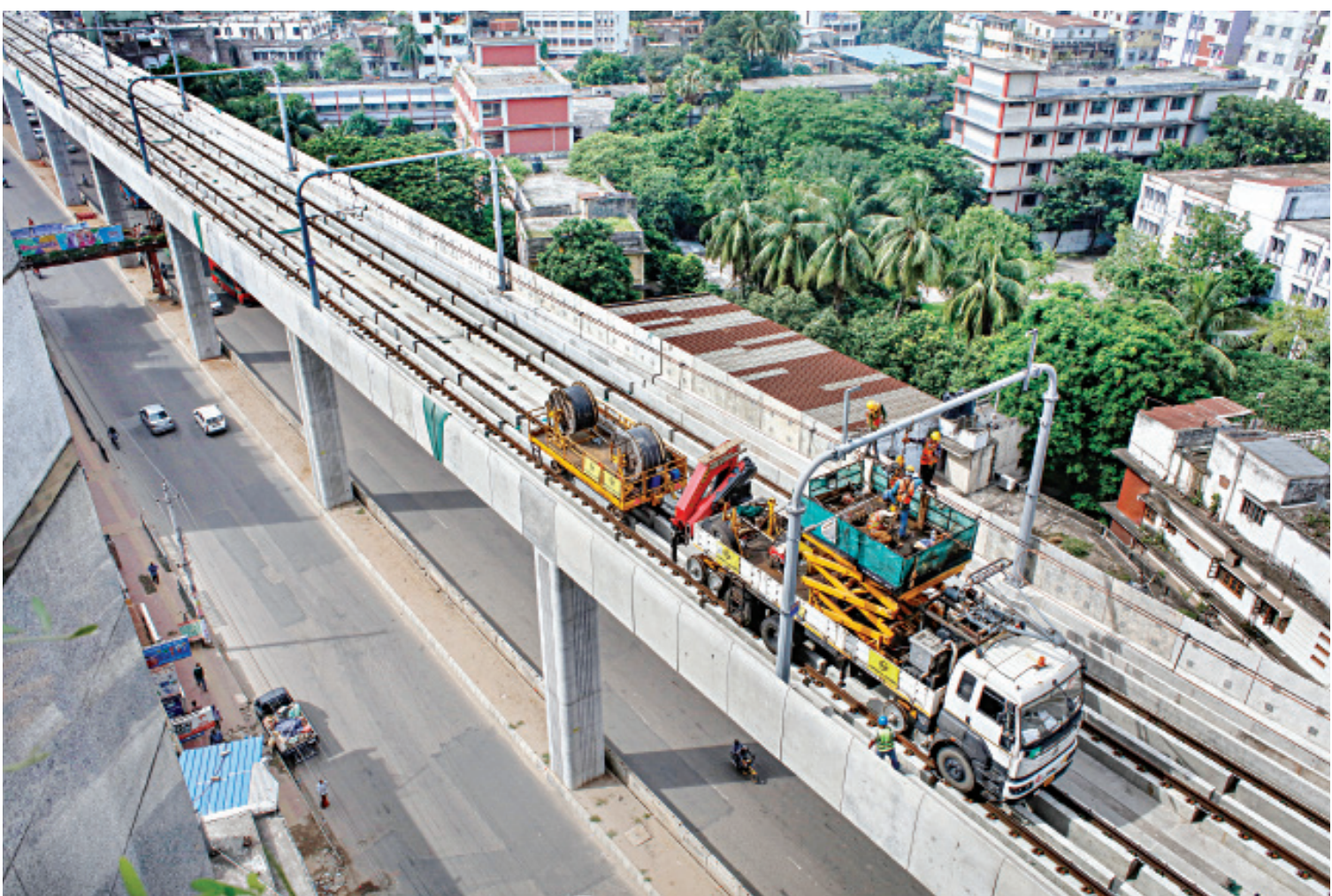
Workers lay out electric lines using a truck, capable of running both on the road and rail tracks, on the country's first metro rail. Construction and installation of different facilities are also nearing completion, with the authorities planning on partially launching commercial operations from December this year. The photo was taken at Farmgate yesterday. PHOTO: RASHED SHUMON
