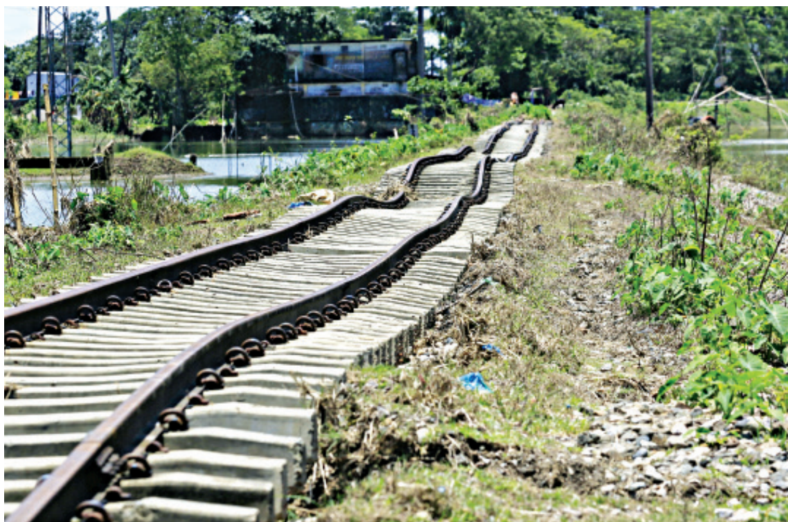
With floodwaters receding in many areas in Sylhet division, a trail of devastation is becoming visible. These rail lines in Chhatak upazila of Sunamganj, which had been under water for days, appear to be warped as the gravel underneath got washed away.
