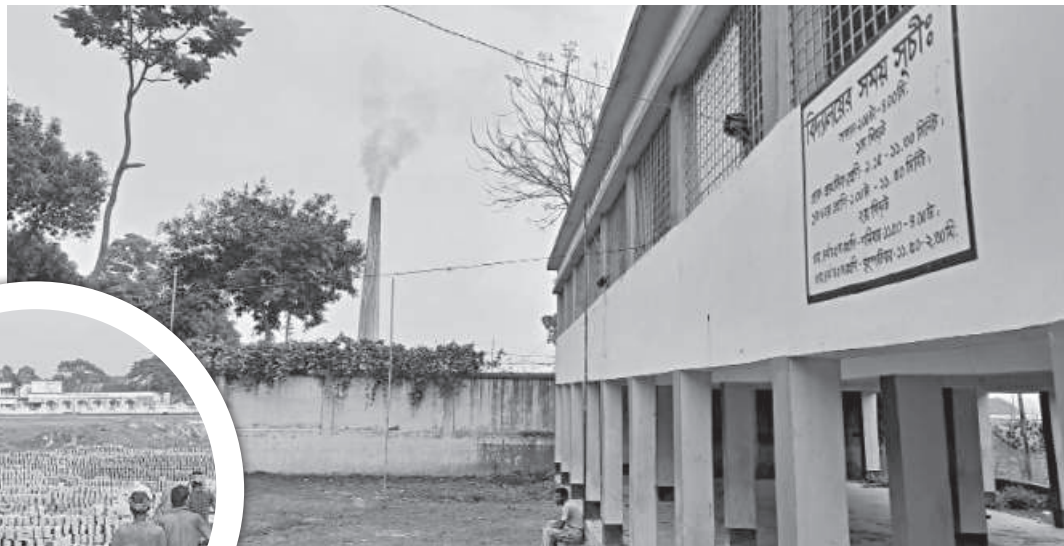
Even though it is illegal to set up brickfields within 1,000 metres of any educational institution under existing law, 17 fields have been set up in close proximity to several schools in Brahmanbaria -- putting almost 10,000 students in the region at risk of health complications.
