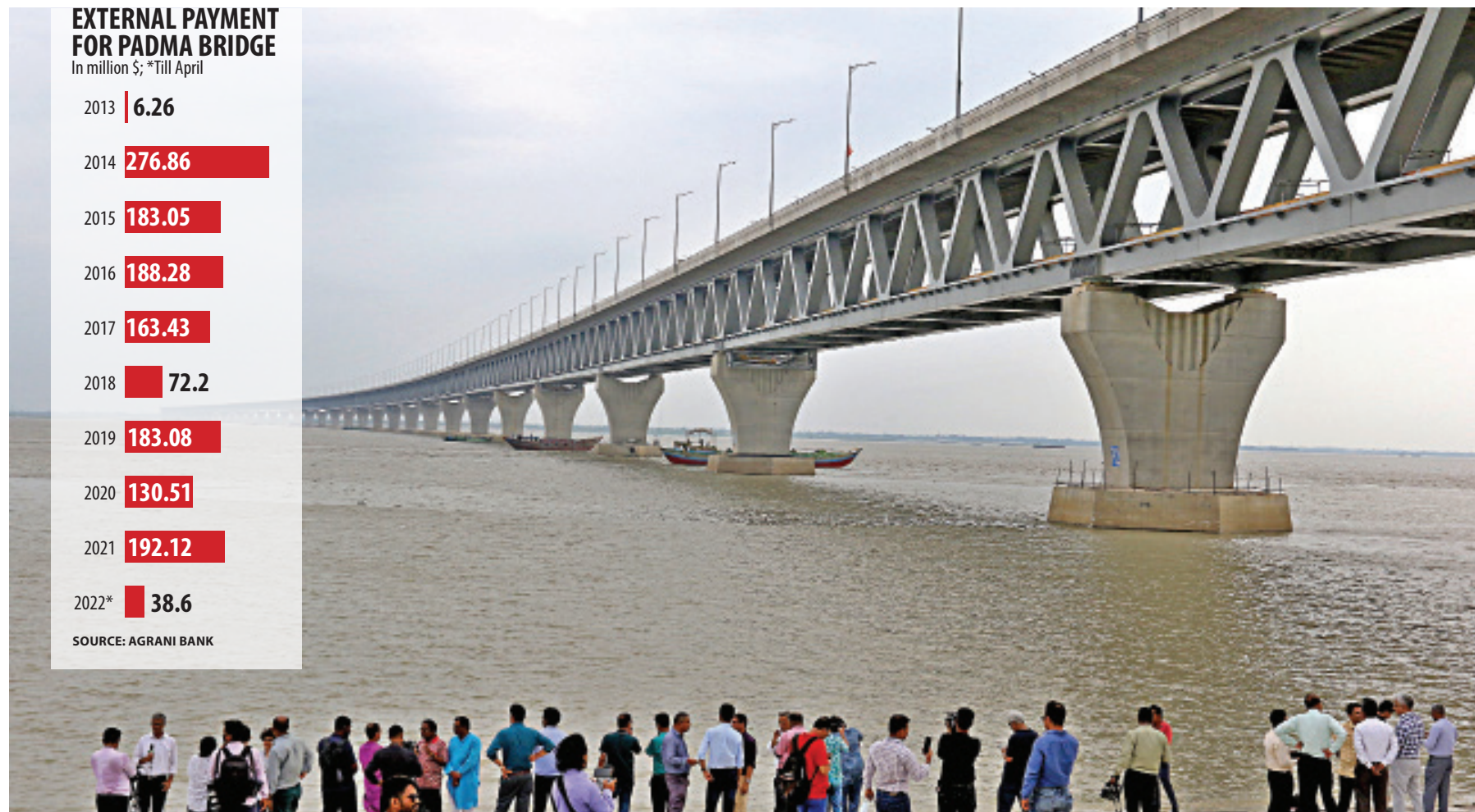
Going on a visit on an invitation of the Prime Minister's Office, journalists soak up the view at one end of the Padma Bridge a couple of days ago. PHOTO: ANISUR RAHMAN
