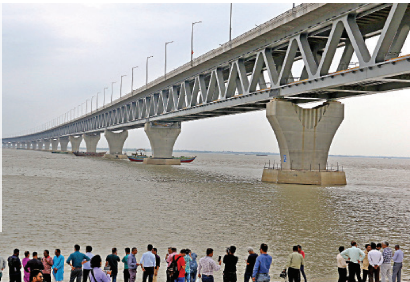
Going on a visit on an invitation of the Prime Minister's Office, journalists soak up the view at one end of the Padma Bridge a couple of days ago. PHOTO: ANISUR RAHMAN
