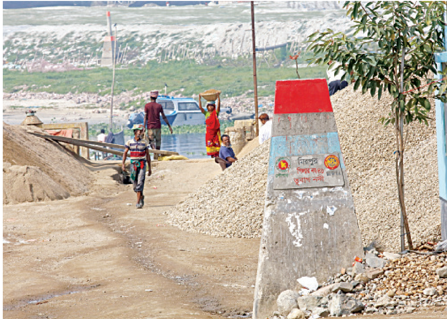
Although BIWTA demarcated Turag River's boundaries, illegal business of construction materials, like sand and stones, was seen booming inside the range. This photo was taken recently from Gabtoli.
