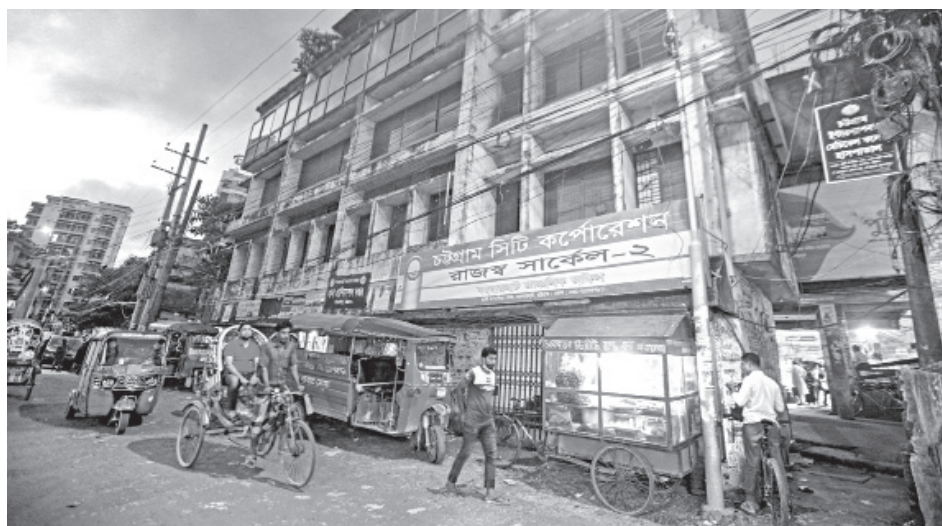
Chattogram City Corporation constructed this building on Chaktai canal's land in 2000 without approval from the development authority. Currently, 47 other illegal structures also occupy the land.
