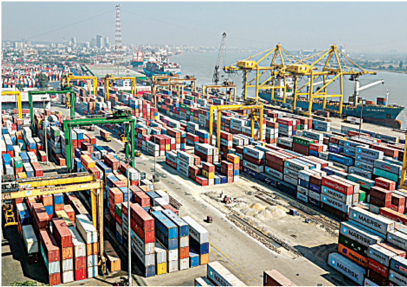
In a bid to reduce the risks of accidents, the port authority is drawing up a set of recommendations for customs authority and port users such as importers, trade bodies, shipping agents and freight forwarders involved in the handling of hazardous cargoes. PHOTO: STAR
