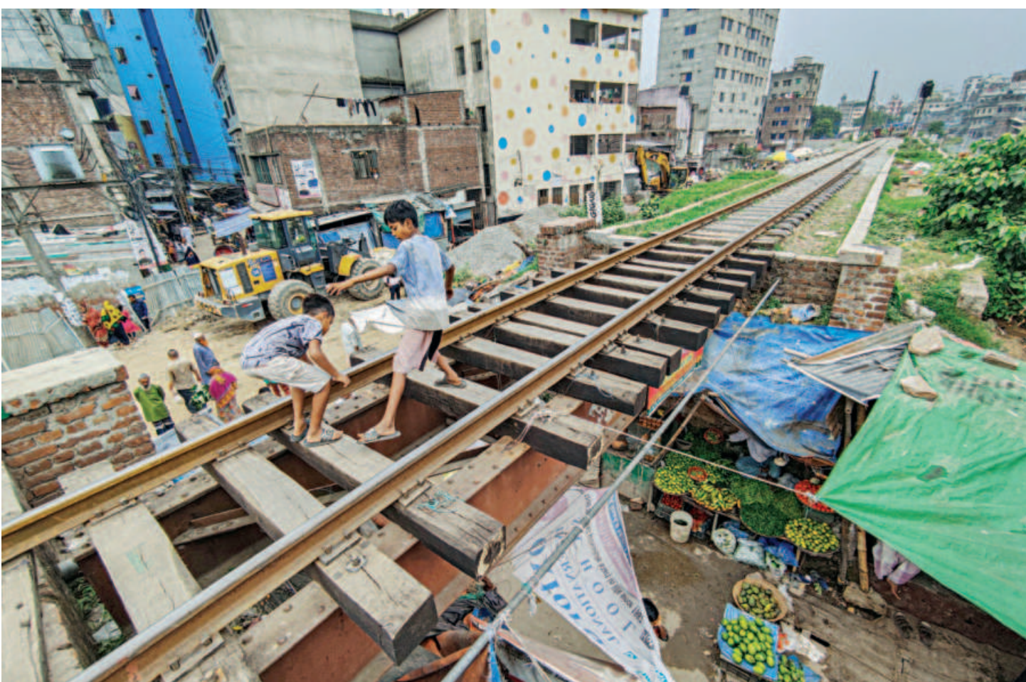
Two children play on a rail bridge over a road in Koratitola in the capital yesterday. If they see an approaching train late, they would not be able to move to the side. They also risk falling to the ground through the gaping openings between the sleepers. Children left to their own devices are often seen on Dhaka streets.
