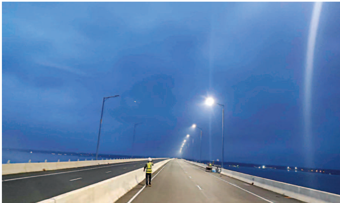
Engineers experimentally illuminating some of the 415 LED lamps that would light up the Padma Bridge once it is inaugurated. The photo was taken yesterday.
