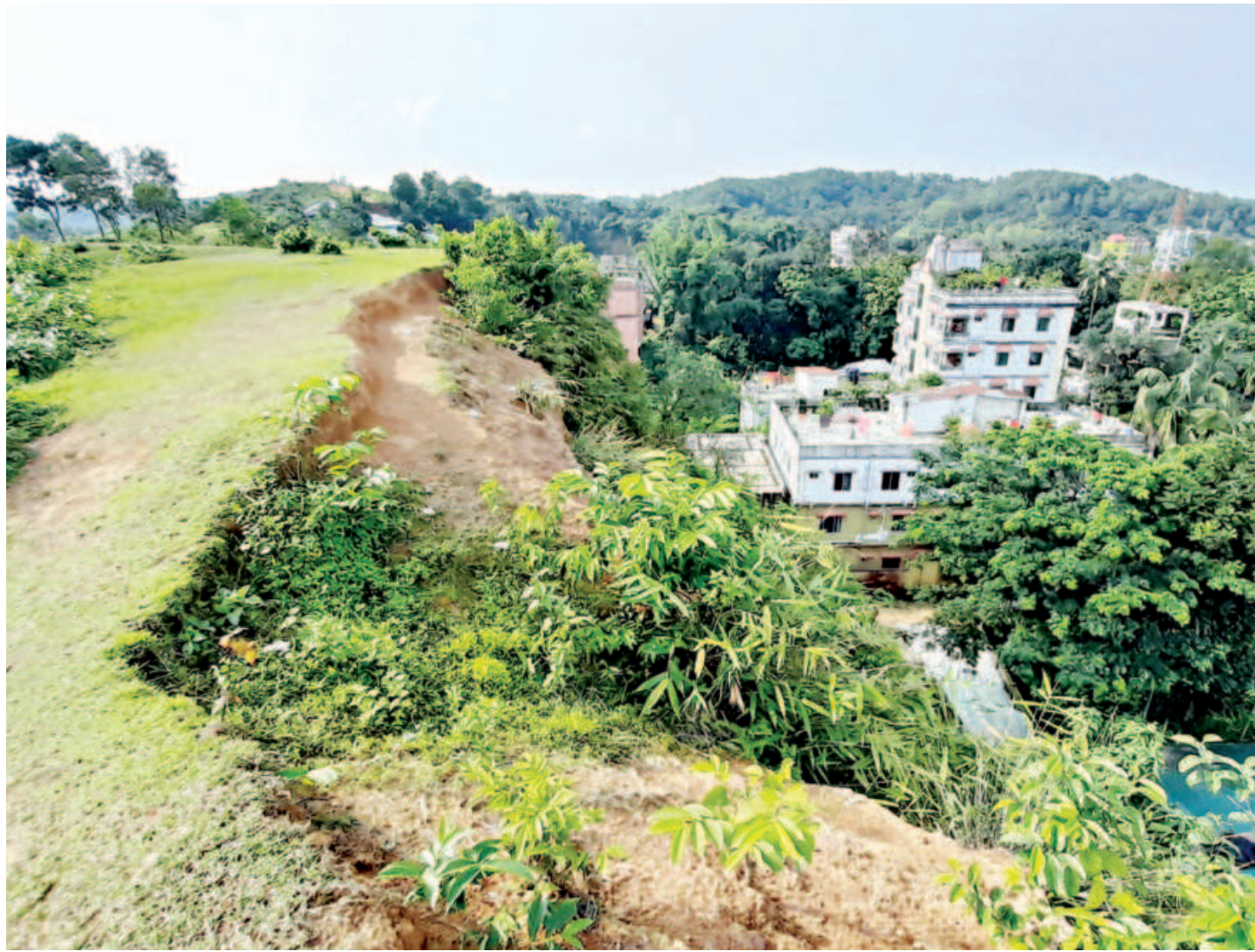
A settlement has been built very close to the steep slopes of a hill in Sylhet city's Akhalia. This exposes the residents of the buildings below to landslides in case of an earthquake or heavy rain. The photo was taken on Wednesday.
