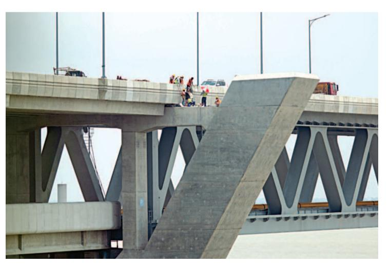
Electricians installing wires to connect one of the 415 lamp posts on the Padma Bridge to the power grid. Work to connect all the lights on the bridge and the approach road could be completed in the next two-three days, and lights on the country's longest bridge may be lit for a trial run by the middle of the month.
